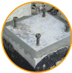
Machine Foundation Grouting
