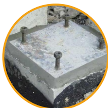
Machine Foundation Grouting
