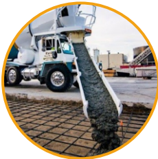
Ready Mixed Concrete
