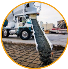
Ready Mixed Concrete
