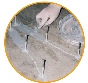
Pipe Joint Filling
