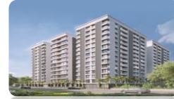
Sheerji Construction, Surat
